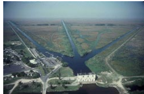
Figure 7. Extensive canal systems and water management have modified the natural hydropattern.
