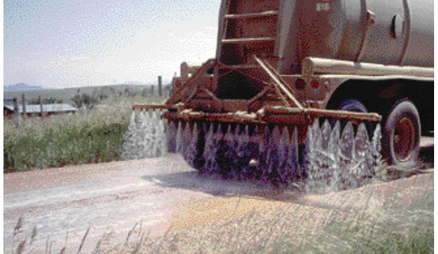
Example of a good piece of application equipment. This truck has a pressurized spray bar with a computerized application system that meters the liquid Chloride with extreme accuracy.
