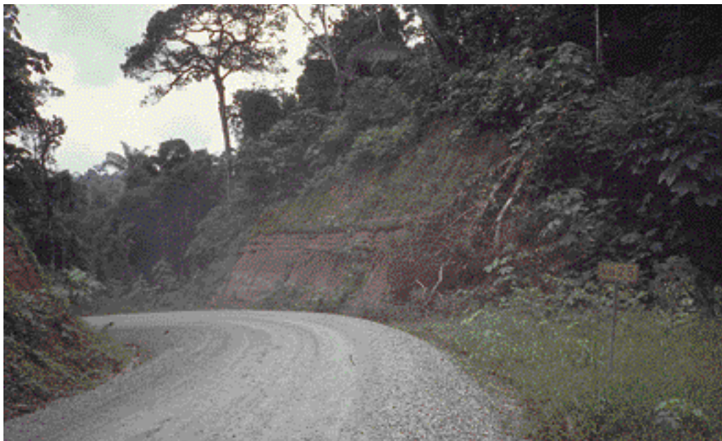
This road in Ecuador has excellent superelevation in the curve. It also has good shoulder drainage and ditches on both sides of the road. (Courtesy of Ron Anderson, Tensar Earth Technologies, Inc., USA)
