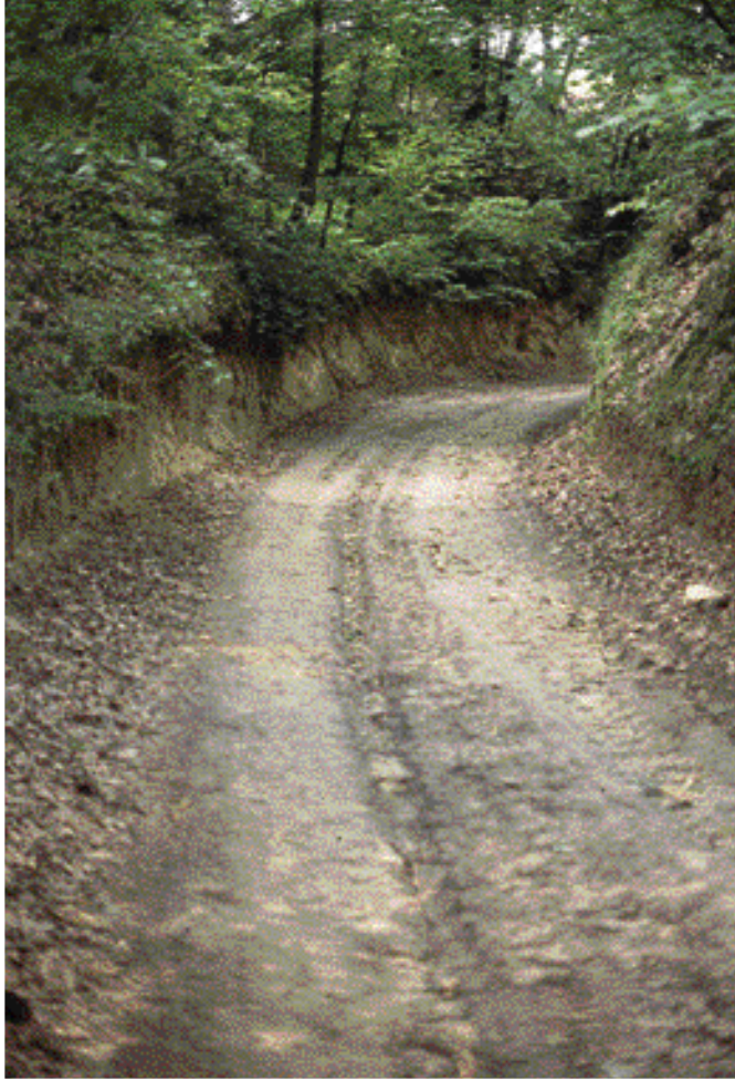
This road, located in Poland, has very poor cross section with no ditches. Consequently, water drains down the roadway itself and after many years of erosion, the roadway is several feet lower than its original elevation. (Courtesy of Mary O'Neill, Office of Remote Sensing, South Dakota State University)
