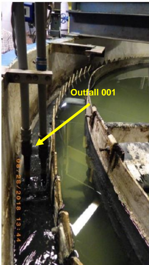
Figure 9 - Wastewater Treatment Clarifier-Outfall 001
