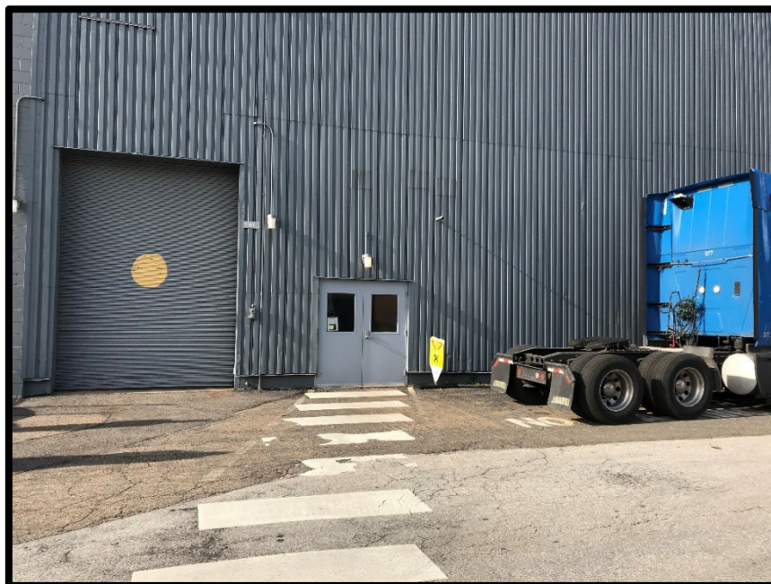
Picture 19: The East wall of building 3-24, which is above the Former Lagoon Area.
