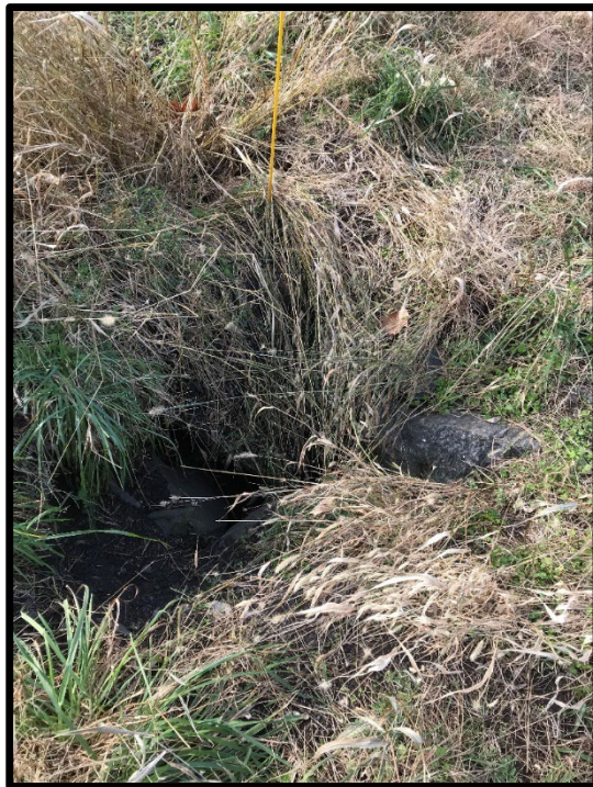
Picture 14: Holes in the Northern edge of Old Landfill Area, facing the south.
