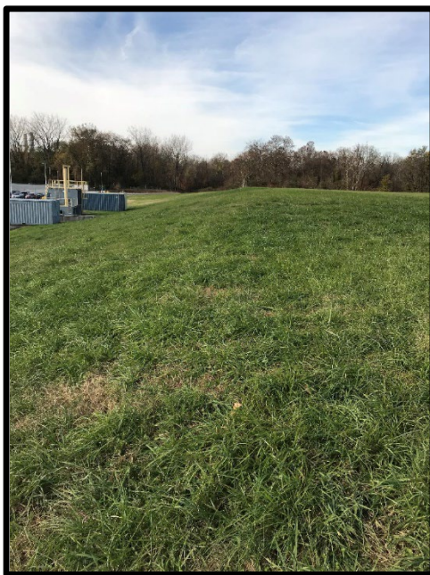
Picture 9: The Sothern boundary of the Old Landfill Area, facing the West.
