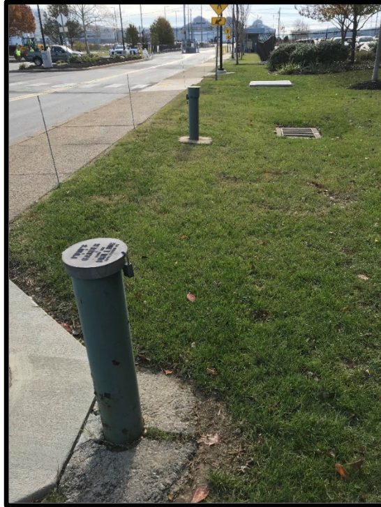
Picture 21: Wells along the eastern edge of building 3-28 facing southeast.
