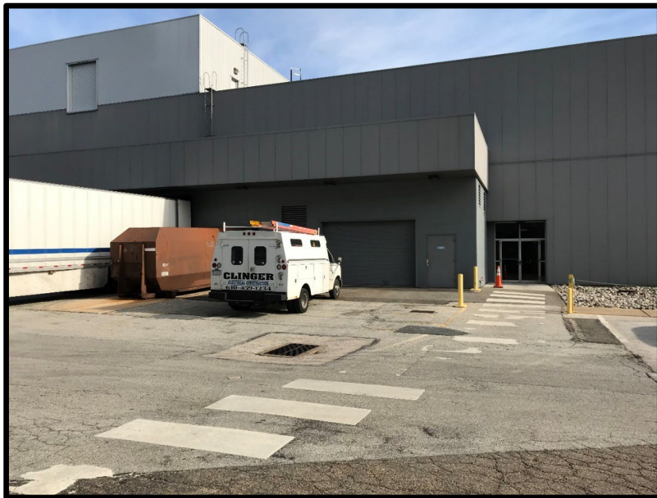
Picture 18: The Western wall of building 3-28 facing the east.
