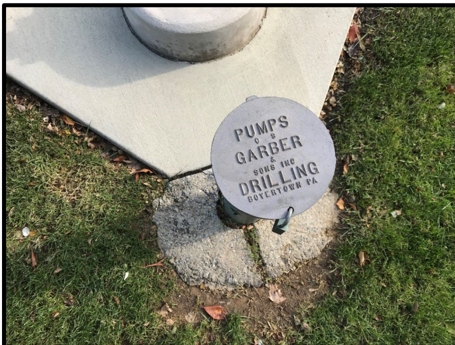
Picture 20: Well located on the east edge of Building 2-38.
