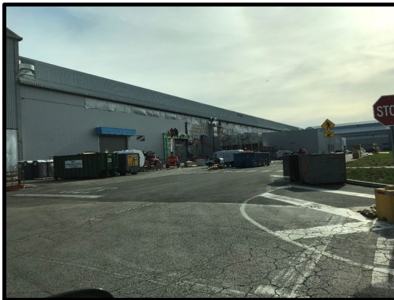
Picture 22: Building 3-57, in southern area, under restoration, facing southeast.
