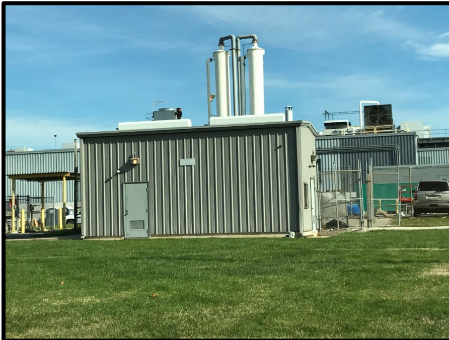
Picture 26: Former ground water pump and treat building, in northern area, currently used for storage, facing east.
