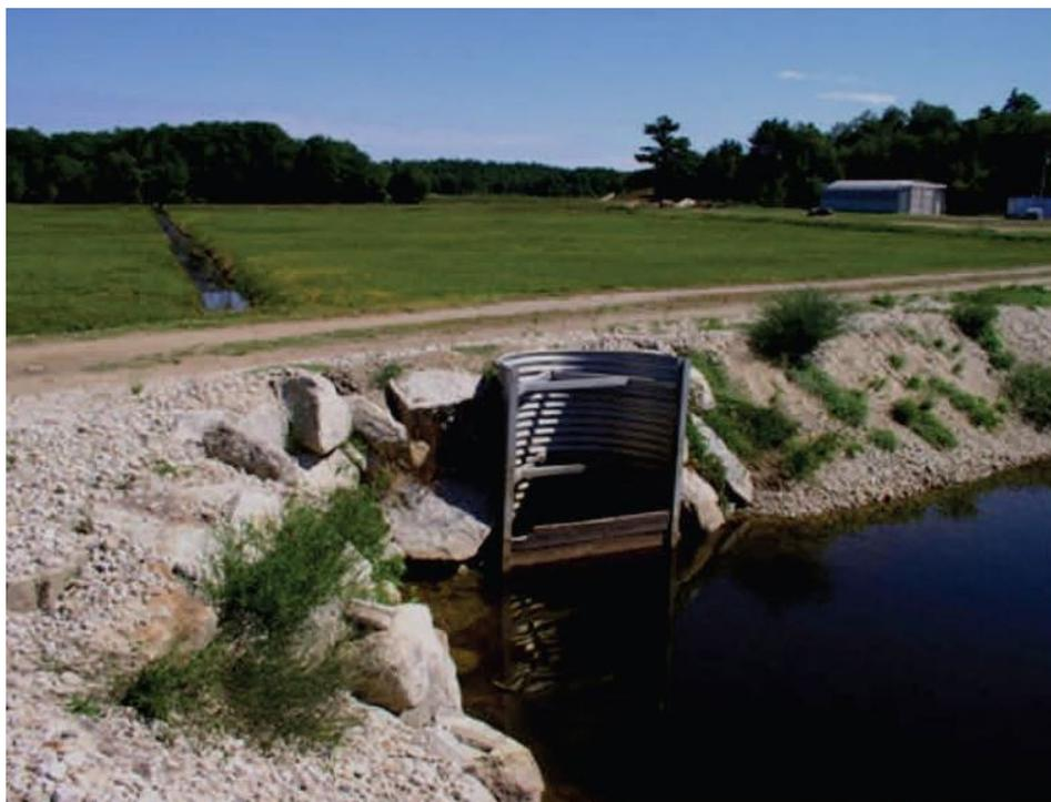
**Figure 5. Controlled Drainage—Example of a flashboard riser. (Source: NRCS 2017a)**
