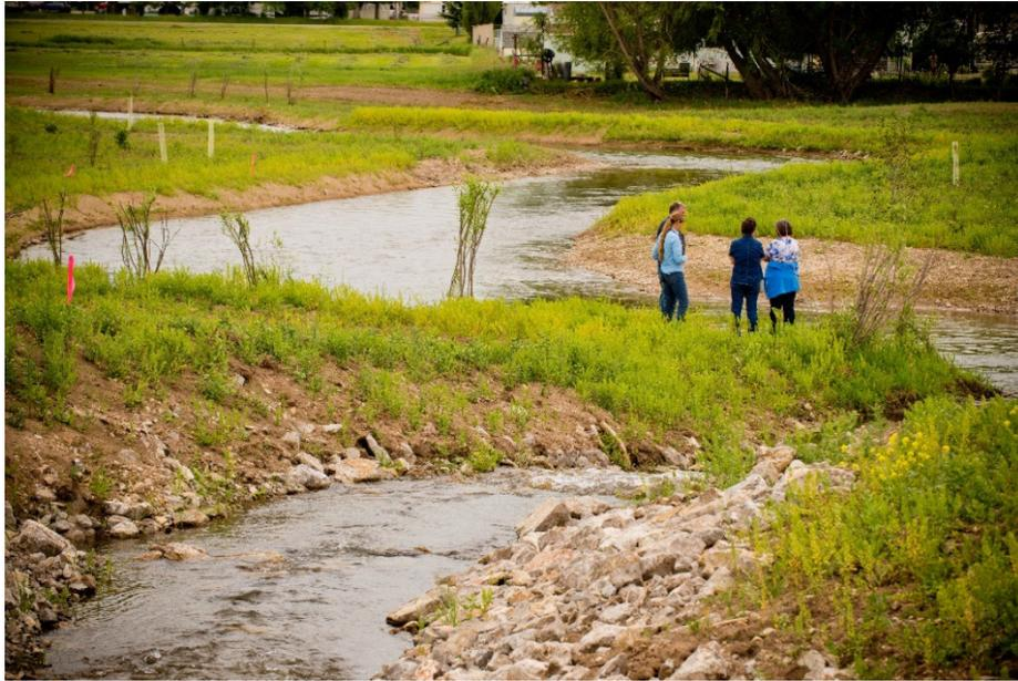
**Figure 7. Streambank Stabilization—Example of riprap banks and channel modifications for channel stabilization and reduced erosion on Big Spring Creek, Montana. (Source: NRCS, Montana 2017)**
