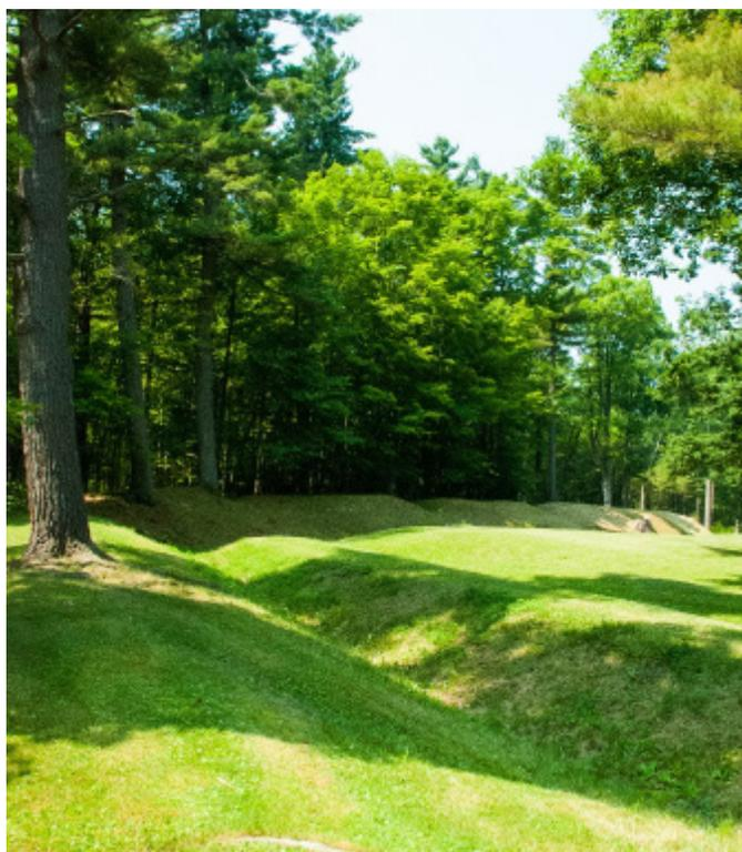
**Figure 14. Grass Swale. (Source: USEPA 2021c)**
