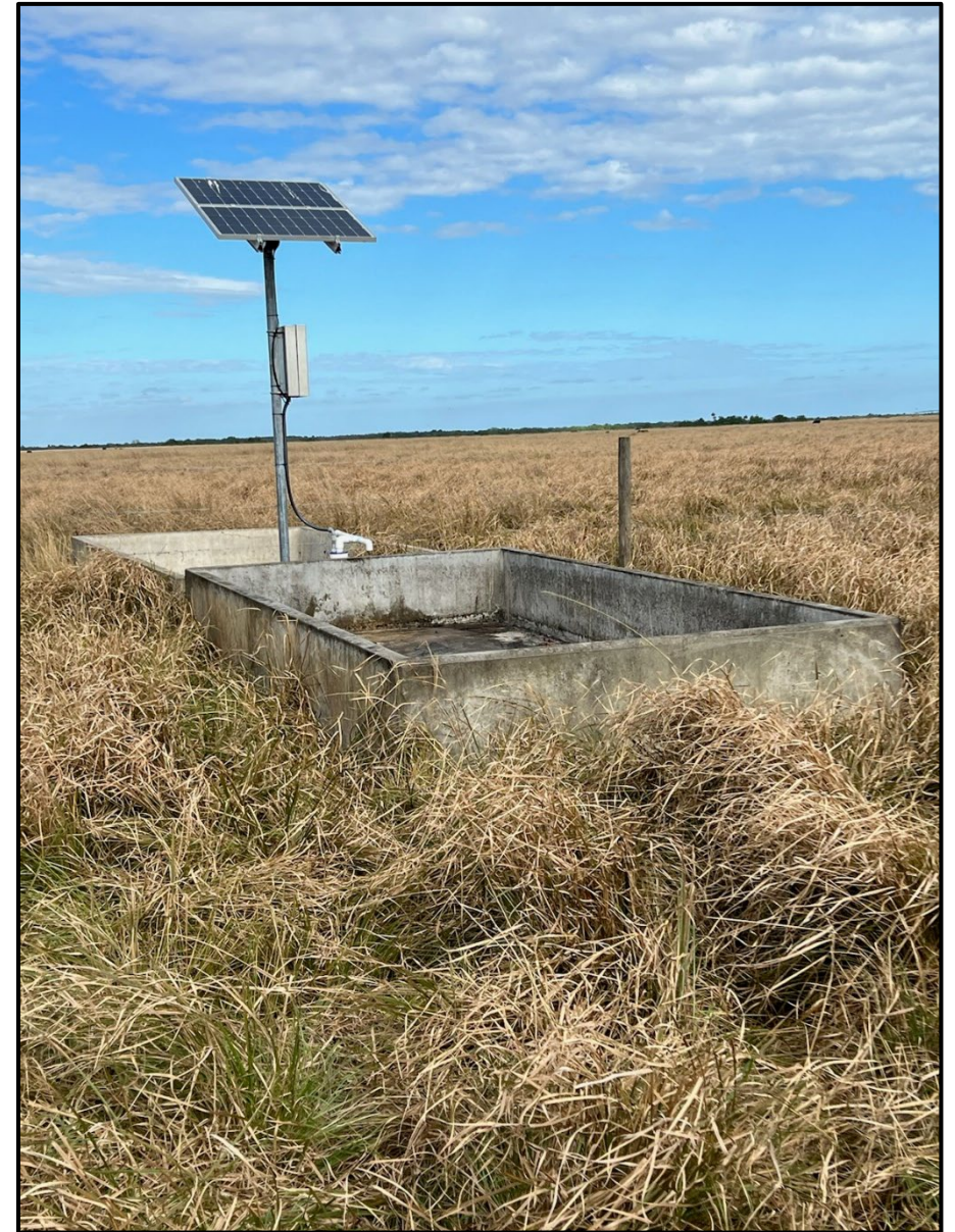
Trough installation with two troughs per solar pump for multiple fields
