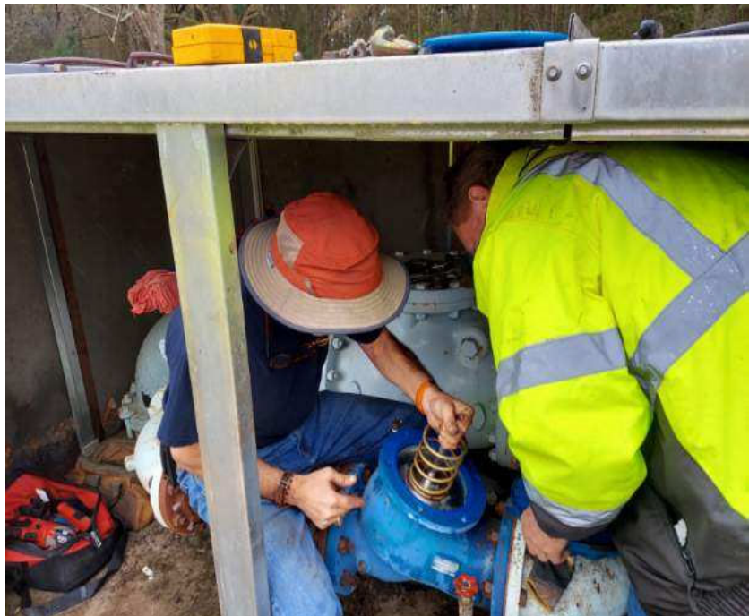
SCRWA staff replacing an altitude valve for Silver Springs Water District in Neeses.
