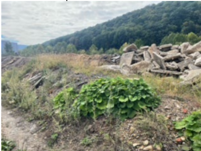
8. Fill material – Oil Valley parcel
