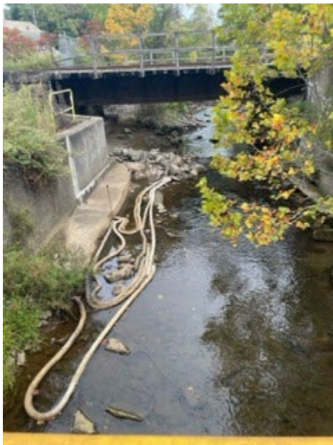
17. Cherry Run bridge and abutment cap remnants– view from walking bridge facing upstream
