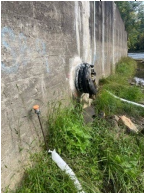
24. Outfall X and typical previous retaining wall fixes
