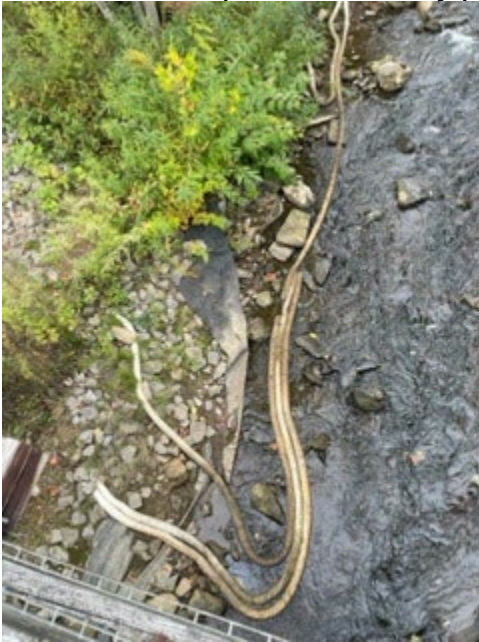
13. Cherry Run abutment cap remnants– looking down from railroad bridge facing upstream
