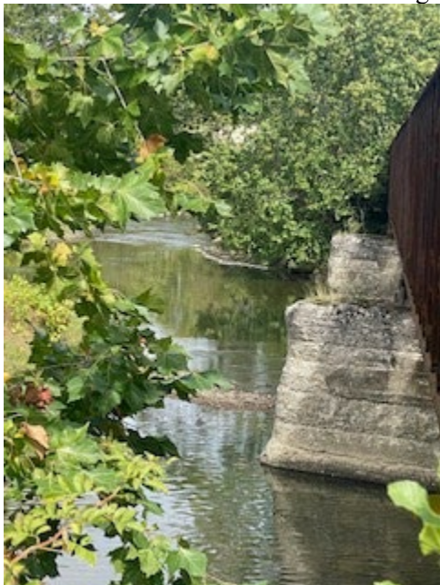
2. Southern End Crude Unloading Area seep - distant
