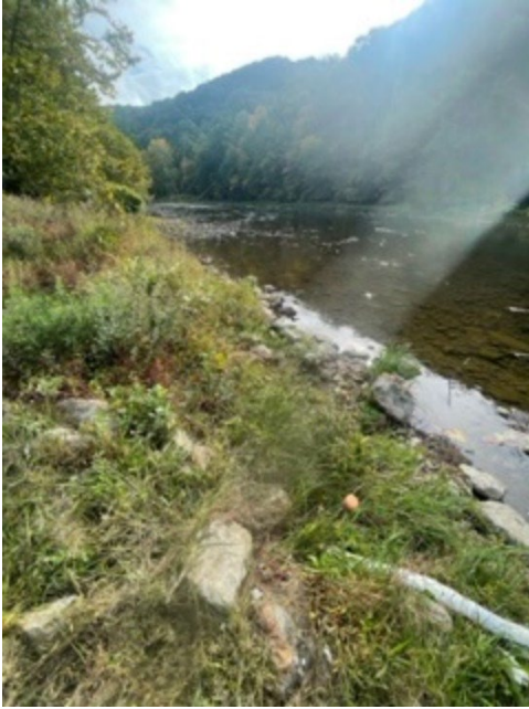
34. top layer restored area (source removal, organo clay, bentomat)
