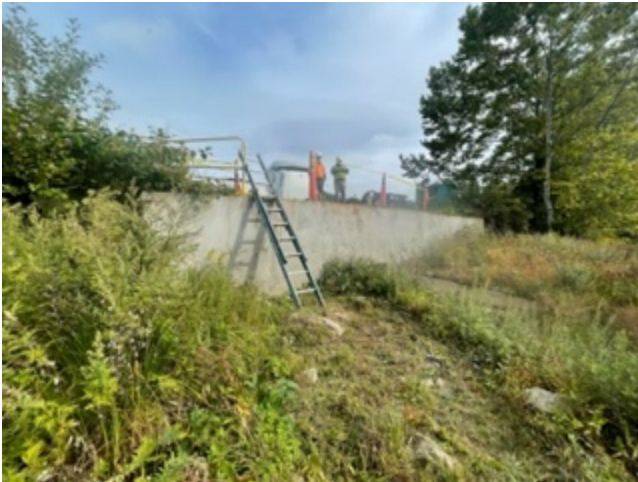
35. shored up crumbling retaining wall in restoration area near pipeyard
