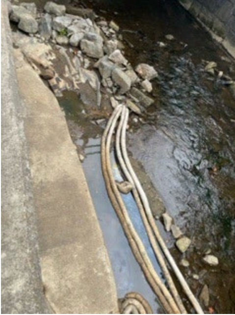
14. Cherry Run abutment cap remnants– at bottom of railroad bridge facing upstream
