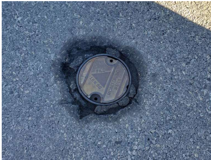
At MW-1A. Monitoring well not labeled with well number.
