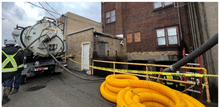
Image 1 – Photo showing vacuum truck and cleaning hose extending into culvert.
