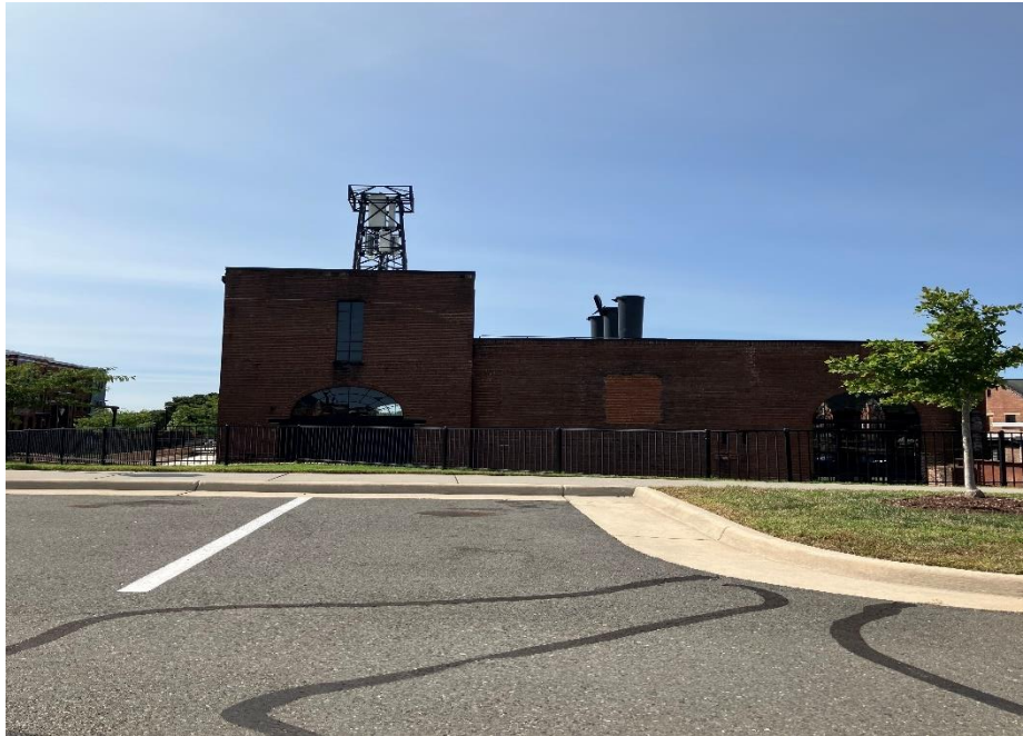
Former clarifier which is still vacant
