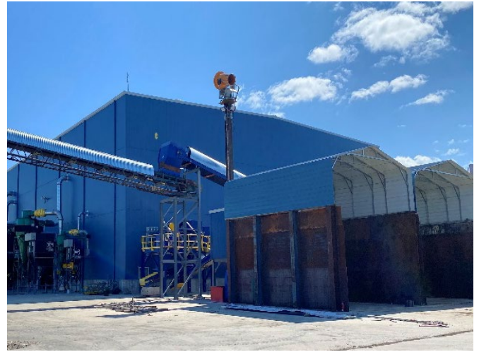
Figure 3: A metal shredding facility with partially enclosed storage bays and a water cannon.
