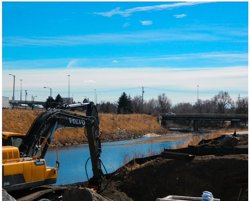
South Platte at Sun Valley during Jetty Construction Photo Credit: Stacey Eriksen
