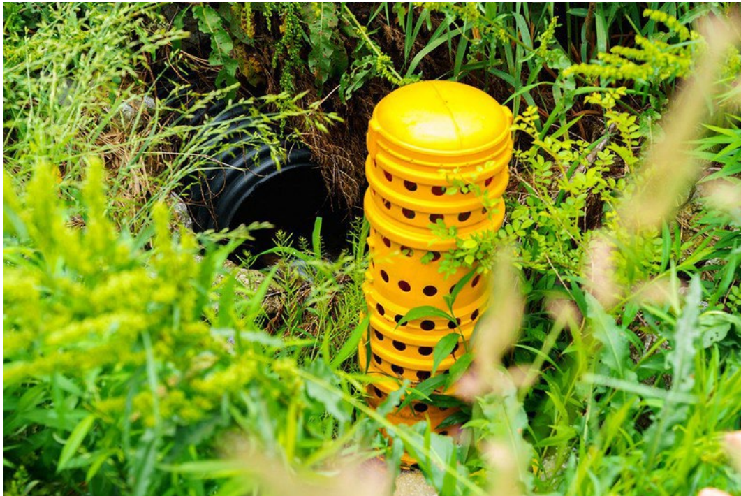
Figure 30. A tile riser inlet allows control of water levels by draining excess water into a tile drain. Photo by U.S. Department of Agriculture.
