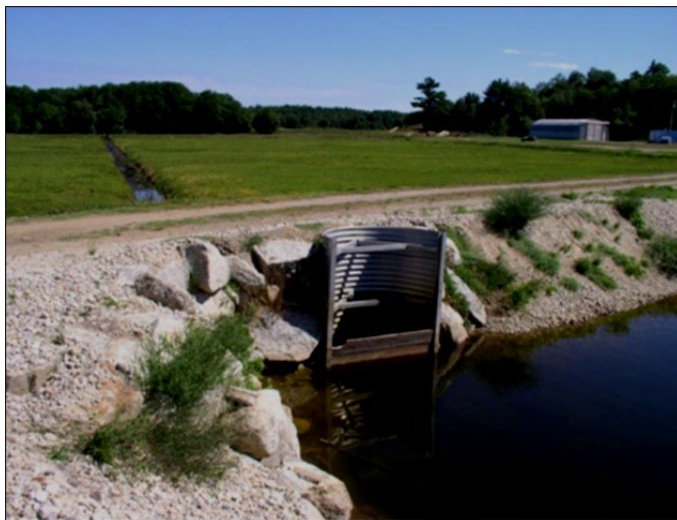
Figure 34. A structure for water control between an irrigation canal and a field with a berm system allows control of water levels in the field. Photo by U.S. Department of Agriculture.
