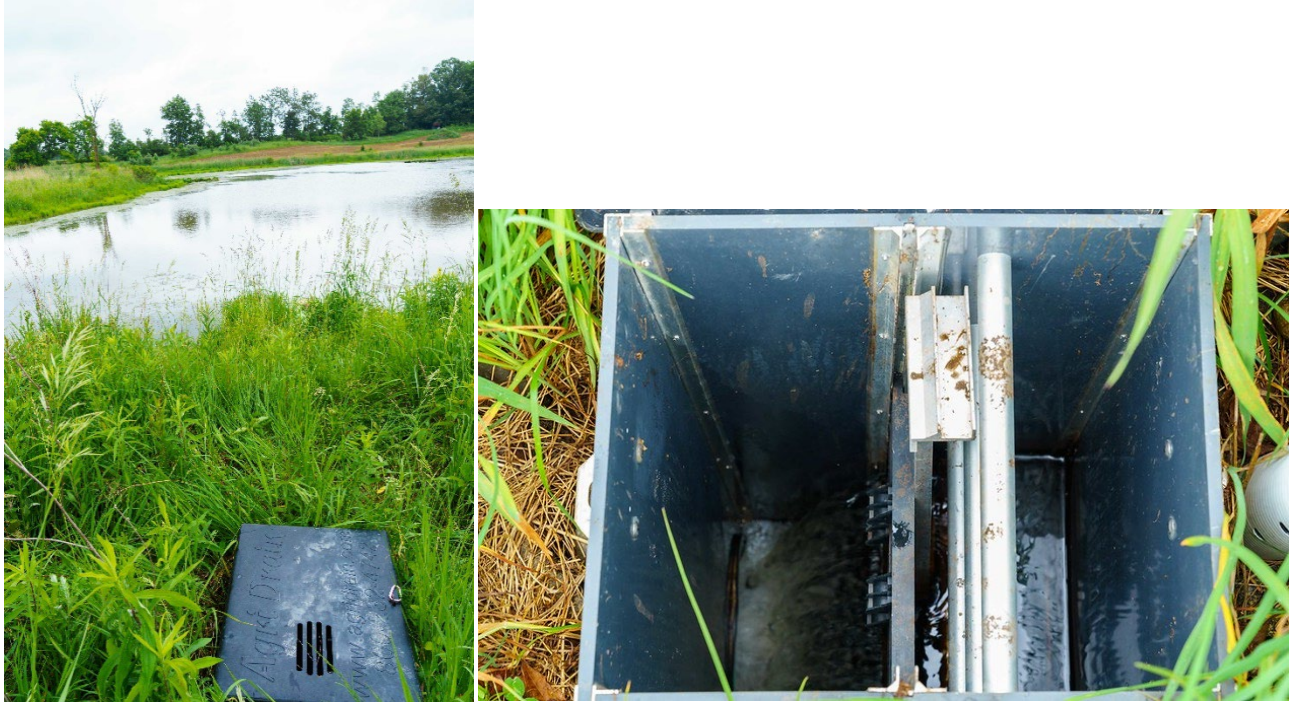
Figure 33. Moving boards inside a water control structure in a wetland in Indiana allow for control of the water level and reduce flooding. Photos by U.S. Department of Agriculture.
