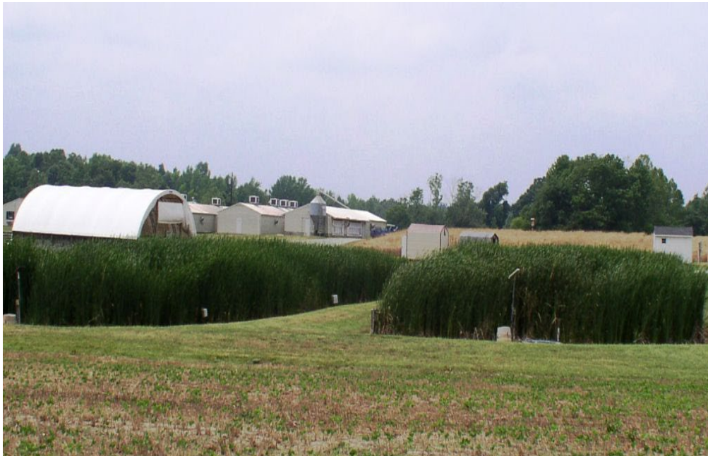
Figure 28. Constructed wetlands on a farm collect runoff from fields. Photo by U.S. Department of Agriculture.
