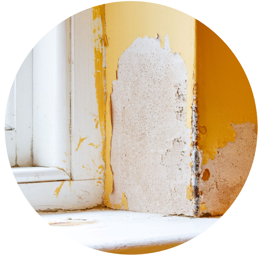
Lead-based paint deteriorates and creates contaminated dust and soil.
