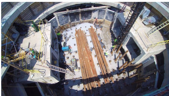
Construction of real-time control project at Hertel Avenue and Deer Street to reduce CSOs by controlling flow to the wastewater treatment plant during wet weather.
