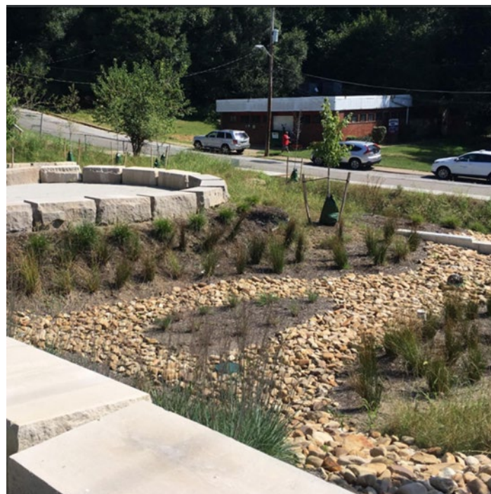
Stormwater BMP installed to meet updated stormwater code requirements.
