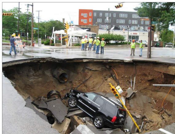
Sinkhole at an intersection after a storm.
